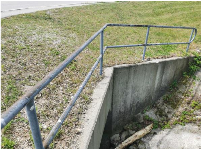
Poor Condition Handrail
