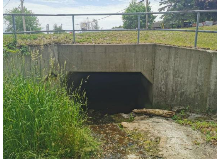
Good Condition Inlet Components
