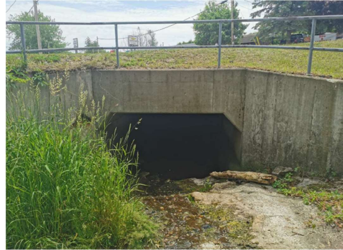
Good Condition Inlet Components
