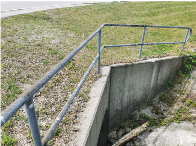
Poor Condition Handrail
